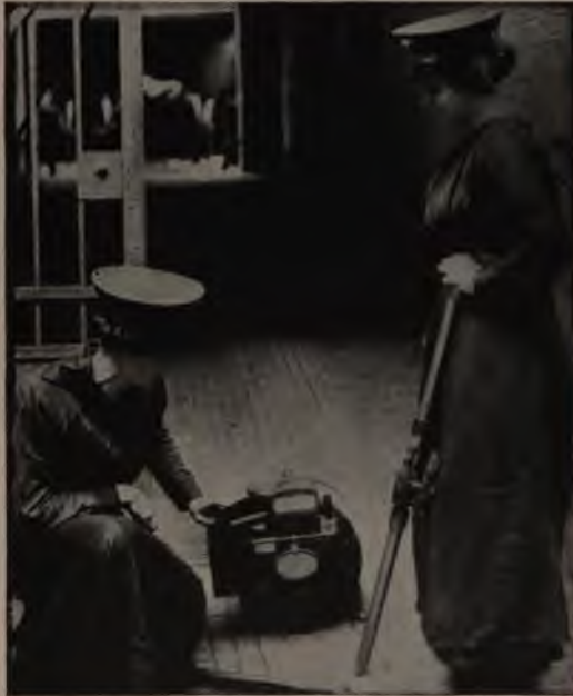
Reading the Gas Meter.
